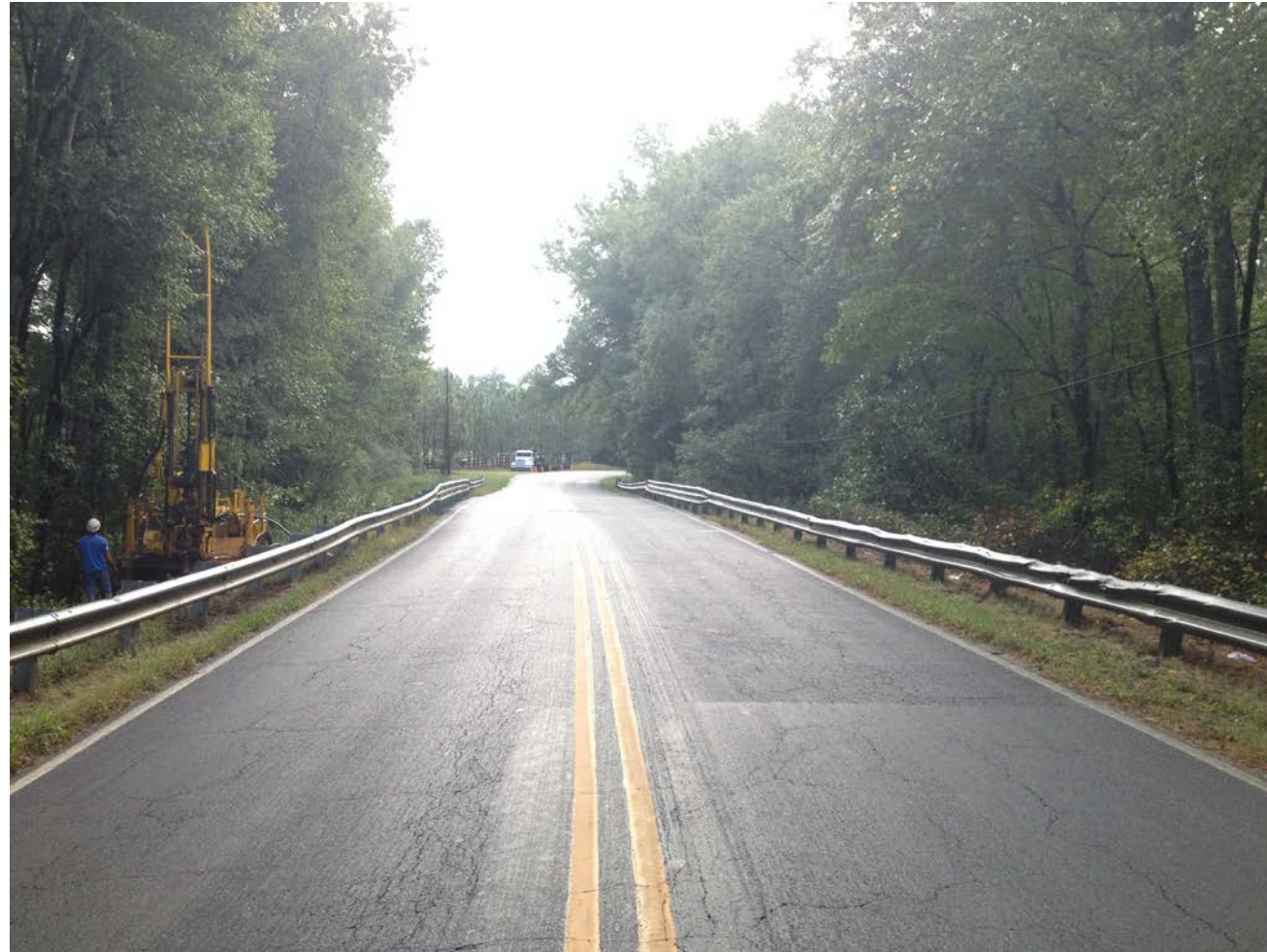
View Facing East (Upstation)
