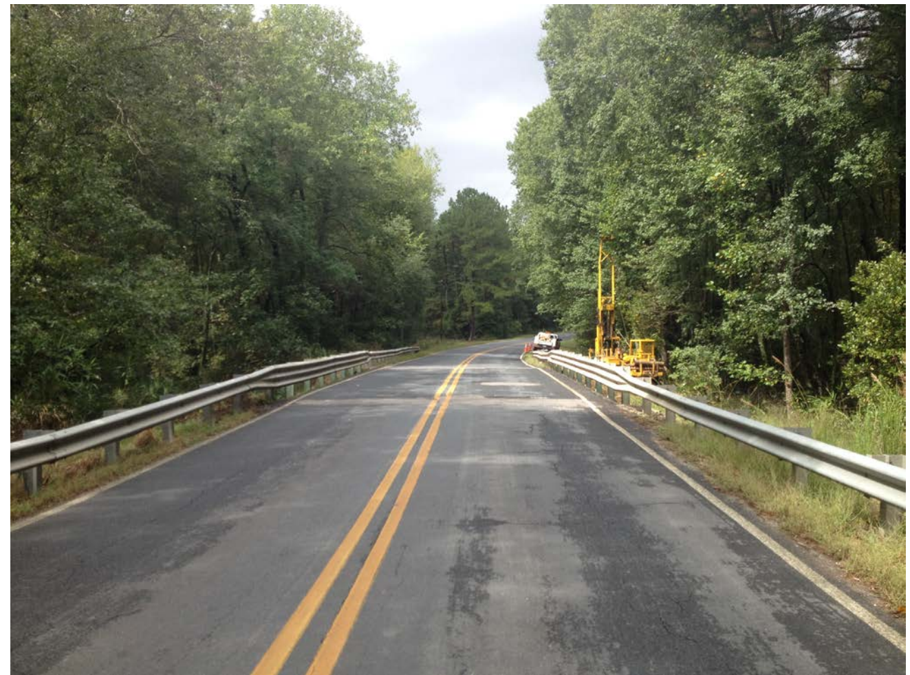
View Facing West (Downstation)
